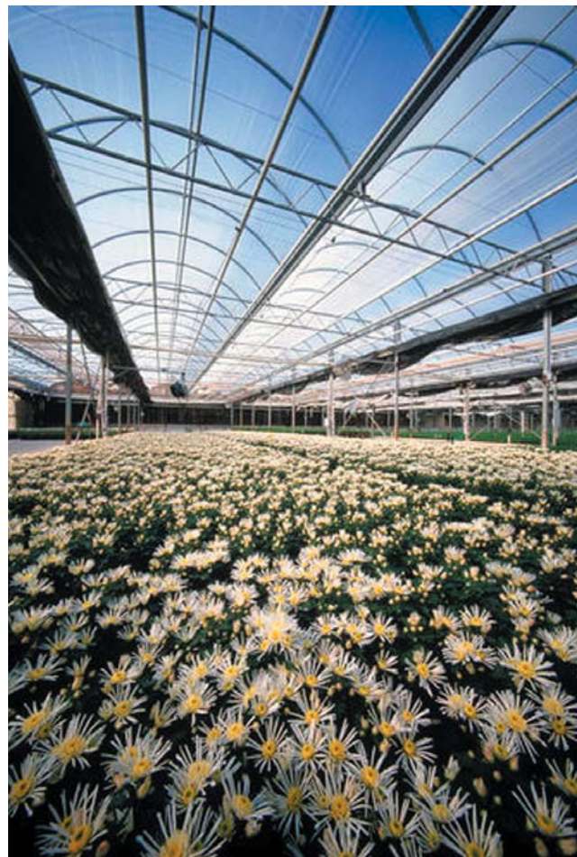
Interior of geothermally heated greenhouse in New Mexico with radiant floor heating, flood irrigation, and overhead curtain for light control.
